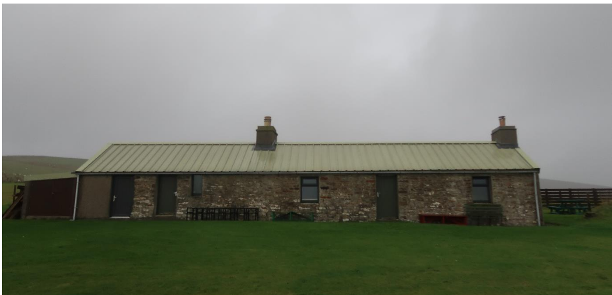
Fig 3: Guides Cottage, front elevation.
